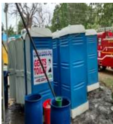
Fig. 3: Zero discharge toilets. However the custom of washing feet after toilet use led to stagnation and mire
